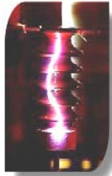
Flashover test of line post-insulator
